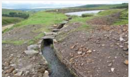
Leat carrying water to a storage reservoir at Nenthead Mines
