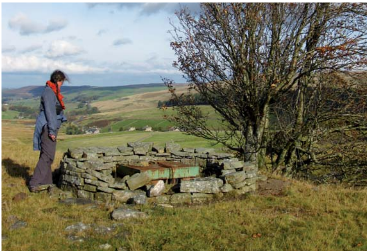
A capped mine shaft west of Allenheads
